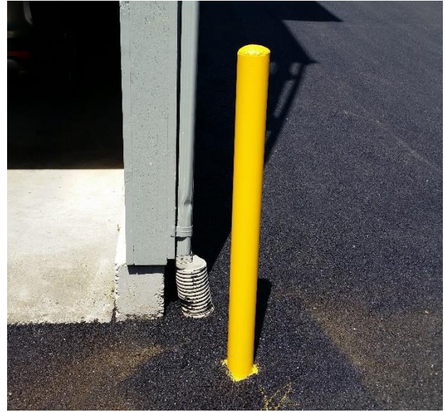
Bollard installed by Lakeside Industries and painted by Quality Coating protects the building wall and downspout against vehicle damage.
