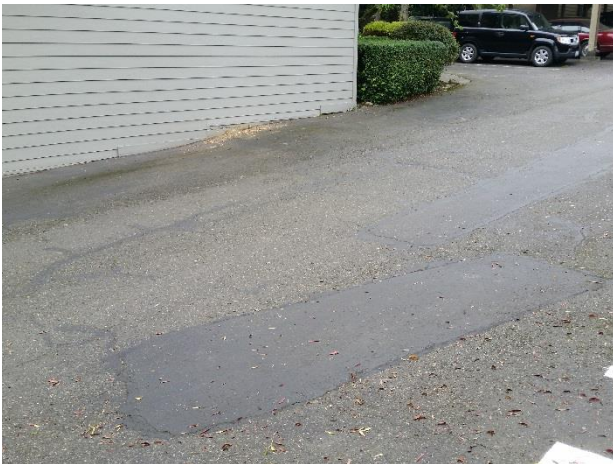
Numerous areas had been patched.
