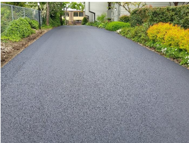
Asphalt completed and includes rolled-up edges to channel water.
