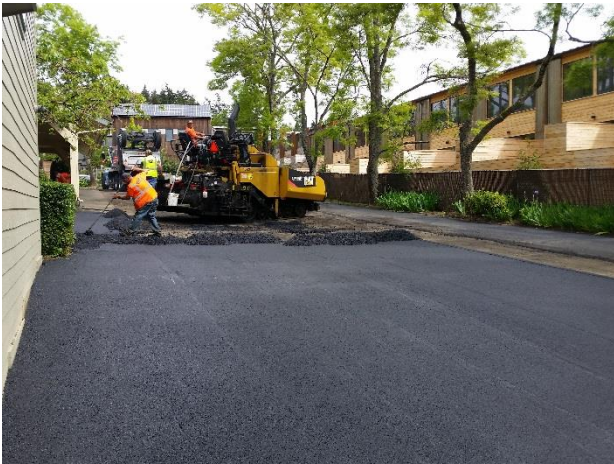
New asphalt installation.
