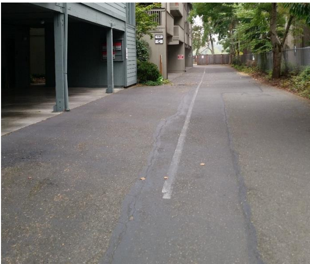
Drain work was completed, leaving additional patches.
