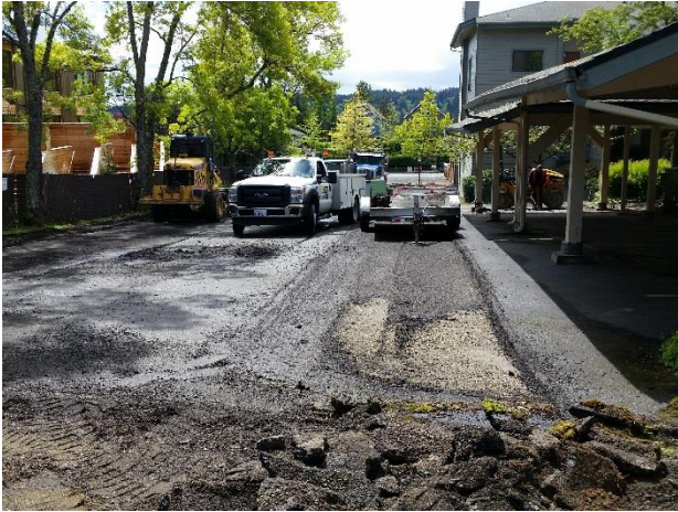
Removal of asphalt.
